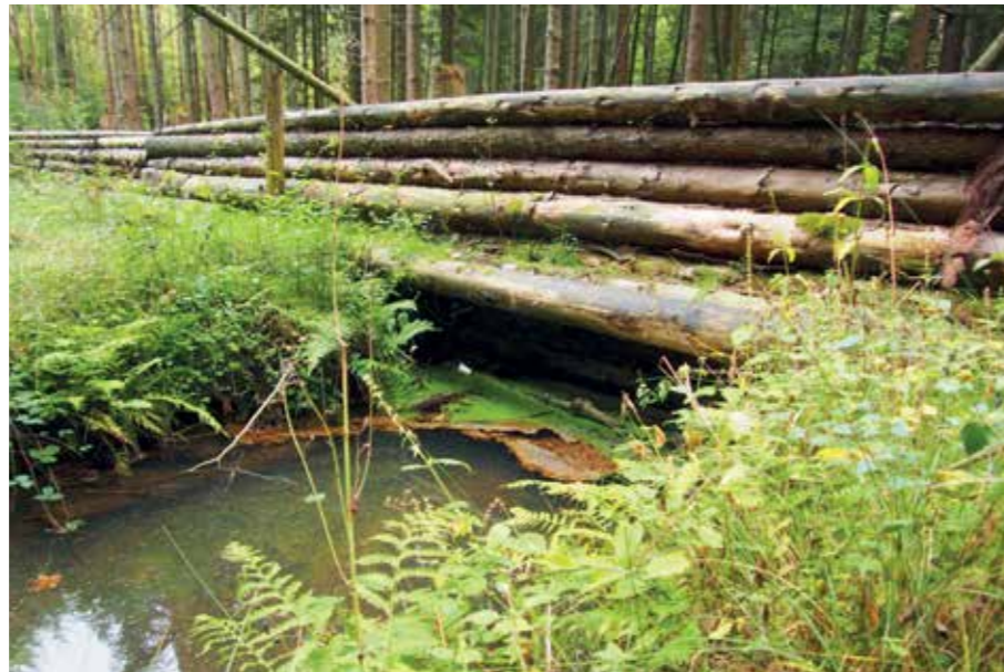
6 – Leaky log dam in the forest above Pickering, England. (Photo: Klára Kerpely, WWF HU)
