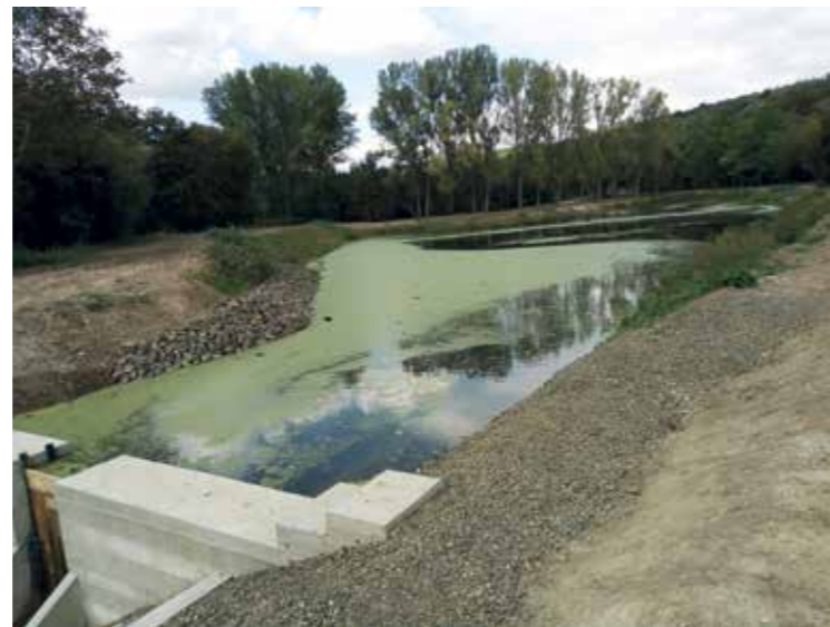
28 – Construction operations in progress in Püspökszilágy. (Photo: The Municipality of Püspökszilágy)
