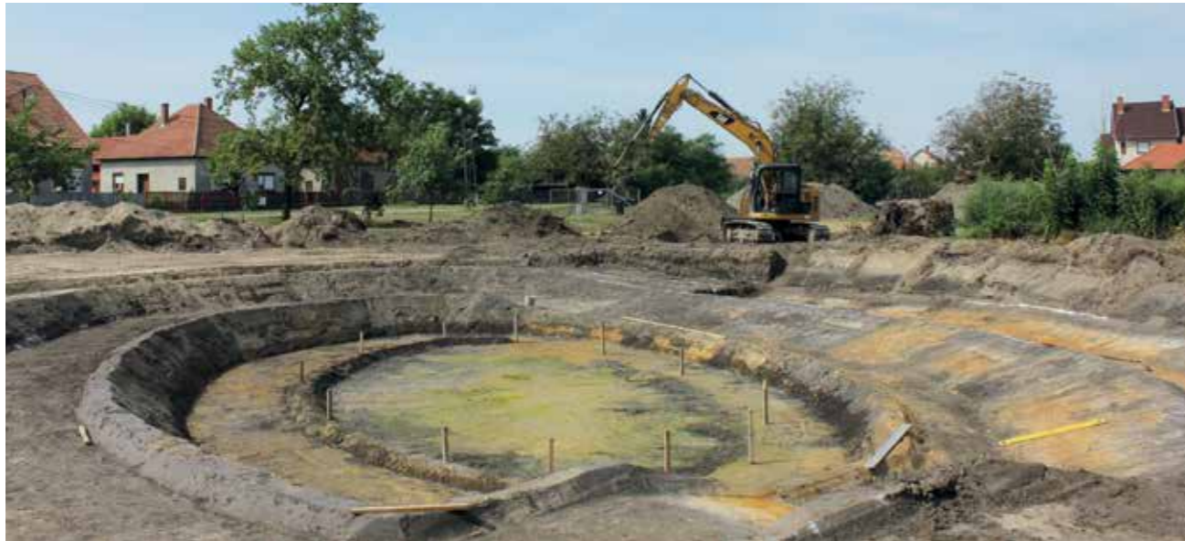
48 – A varied irregular basin geometry created in Ruzsa. Flat slopes and stepped embankments were built in alternation, taking closer attention and work on the part of the contractor and even reducing the volume of the reservoir in comparison with one with the steepest possible slope. A less steep bank however, is both safer and makes a more versatile habitat for aquatic wildlife. (Photo: V. Mátyás Farkas, HU)
