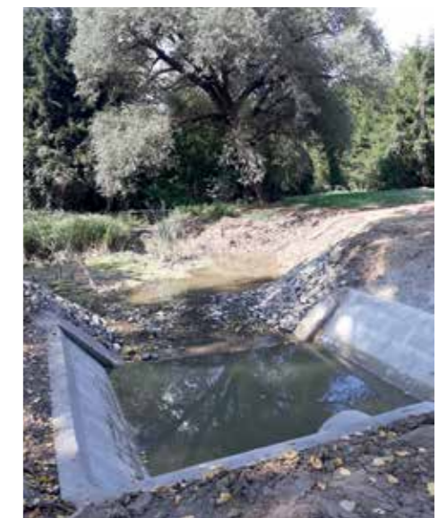
50 - Construction of sediment traps for the Püspökszilágy storm water reservoir (Photo: Viktor Mátyás Farkas, WWF Hungary)
