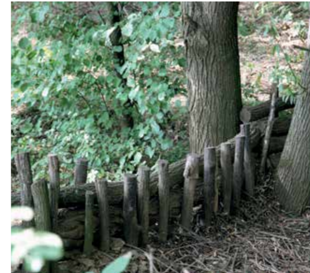
29 – Log dams at Püspökszilágy during the dry period, and “at work”. (Photo: Ministry of Interior, Püspökszilágy Municipality)
