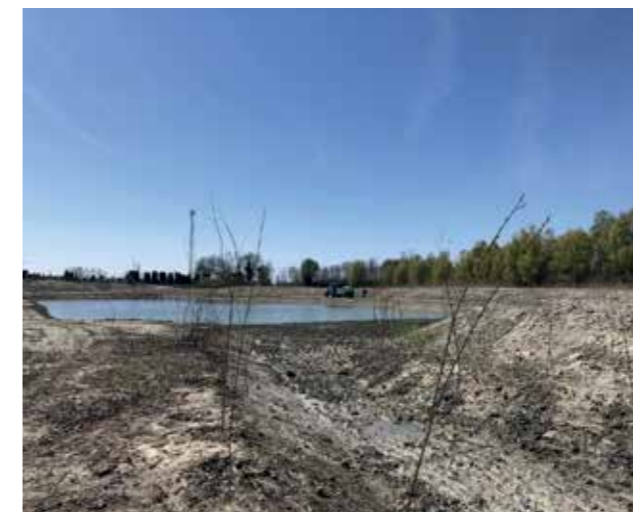
20 - Earthworks in progress in the village of Bática. (Photo: Zsófia Szabó, Bática)
