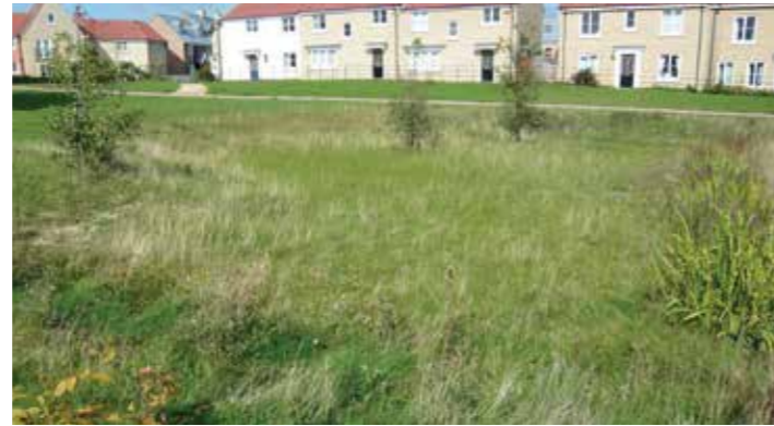
11 – Storm water reservoir suitable for temporary inundation, also functioning as a green surface. (Source: susdrain.org)
