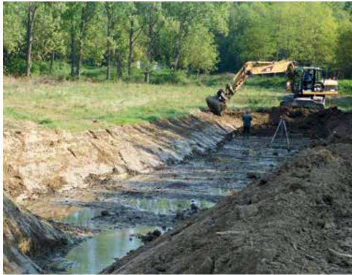
27 – Works in progress in Püspökszilágy. (Photo: the Municipality of Püspökszilágy)
