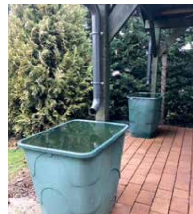
13 – A simple and inexpensive rainwater collecting system for retaining and utilising rainwater around the house. (Photo: Zsófia Szabó, Bátya)
