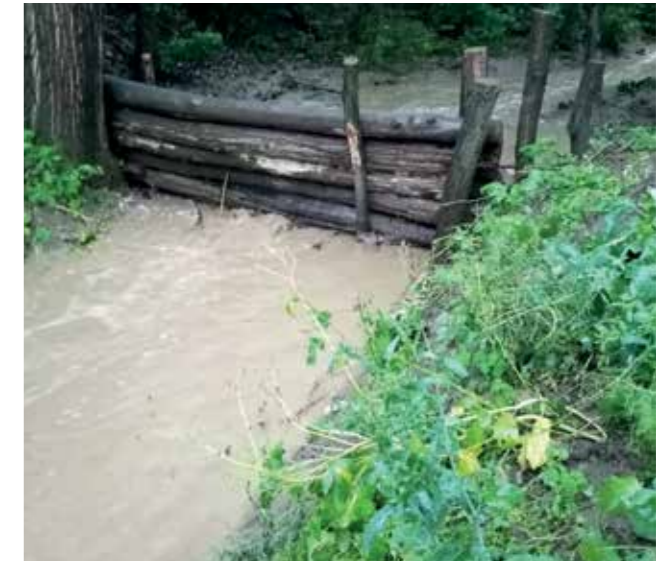
29 – Log dams at Püspökszilágy during the dry period, and “at work”. (Photo: Ministry of Interior, Püspökszilágy Municipality)
