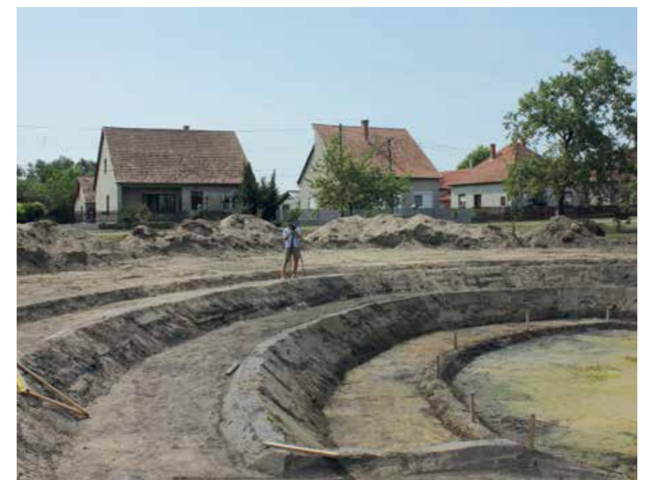
33 – Shaping a varied lake bed surface for the local pond at Ruzsa. (Photo: WWF)
