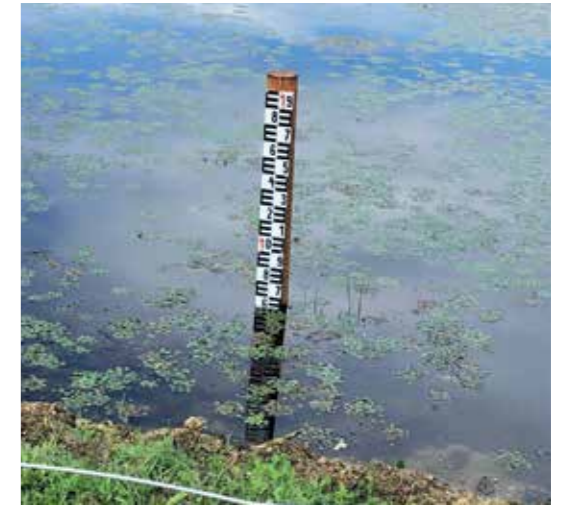
43 – Installed water level gauge at Tiszatarján. (Photo: the Municipality of Tiszatarján)
