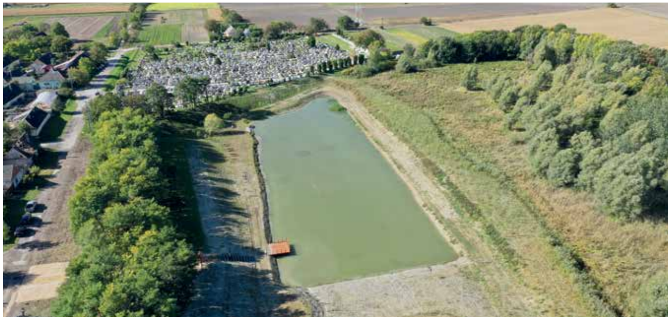
23 – The finished project: two-basin open-surface reservoir pond. (Photo: Filmever Stúdió)
